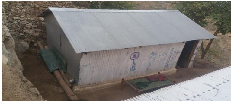
Figure 21: A shelter provided to earthquake affected family in Shangla District (Photo Credit: GLOW)
